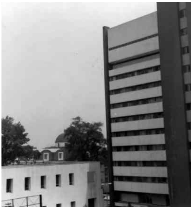
Torre del Hospital Juárez
